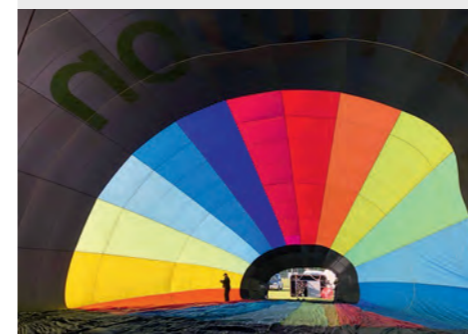
Balloon envelope inspection
